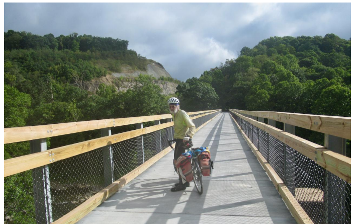
One of the longer, railroad trestles on the GAP trail
