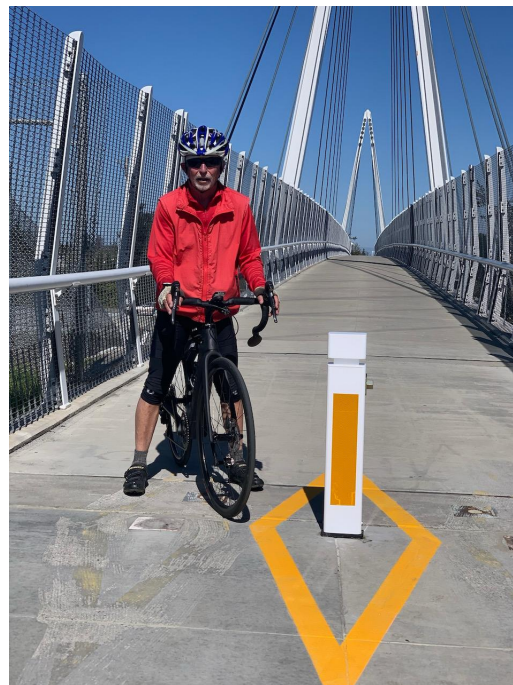
Pete next to the highly visible, single bollard on the Don Burnett Bridge entrance
